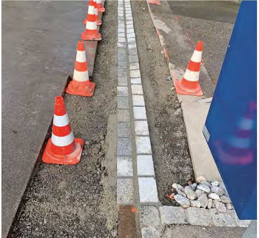
Randstein Reparatur Wingerstrasse, Salez
